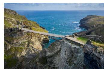
Footbridge in Tintagel Castle, Tintagel, United Kingdom. William Matthews associates + Ney & Partner
