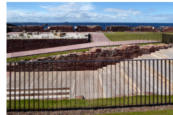
The Dunbar Battery, Dunbar, Scotland, United Kingdom. rakinfraser landscape architecture
