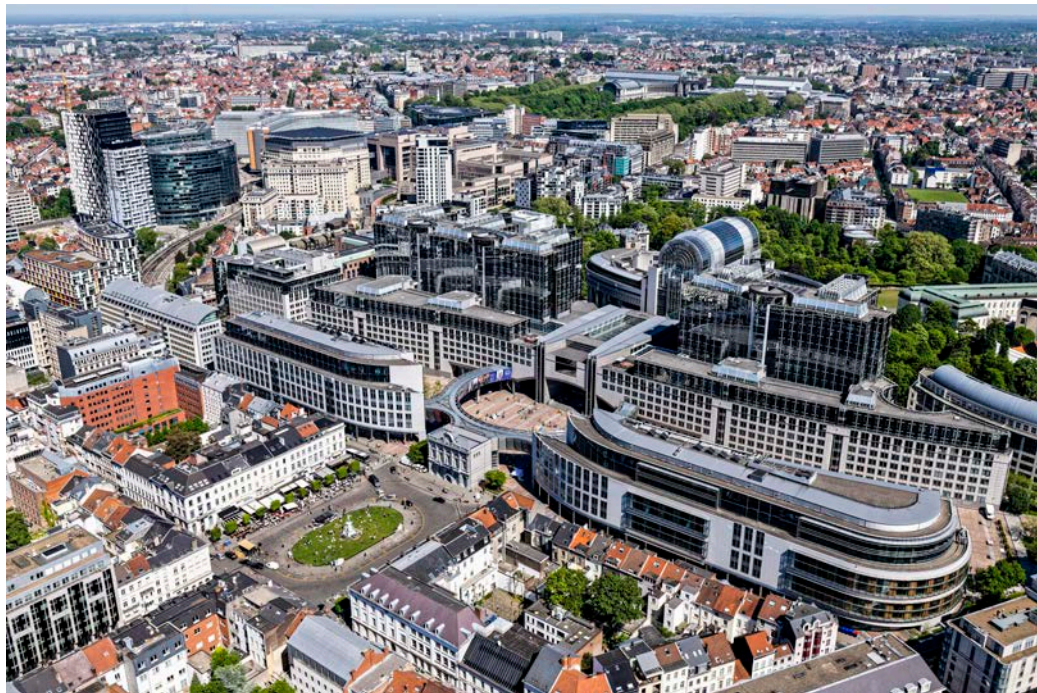
Figure 4: View of the Paul-Henri SPAAK Building with Parc Léopold in the background and Place du Luxembourg in the foreground, © Façade and hemicycle: architect Michel Boucquillon).
